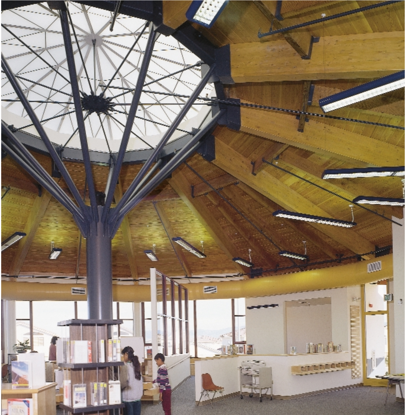
Lincoln School in Spreckles, California is home for the local county library where Alaska Yellow Cedar and Douglas-fir glulam members add light and warmth.
