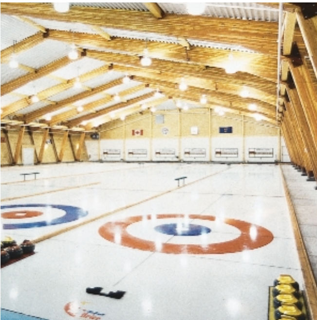
Glulam cantilevered frame for curling rink, Calgary, Canada.
