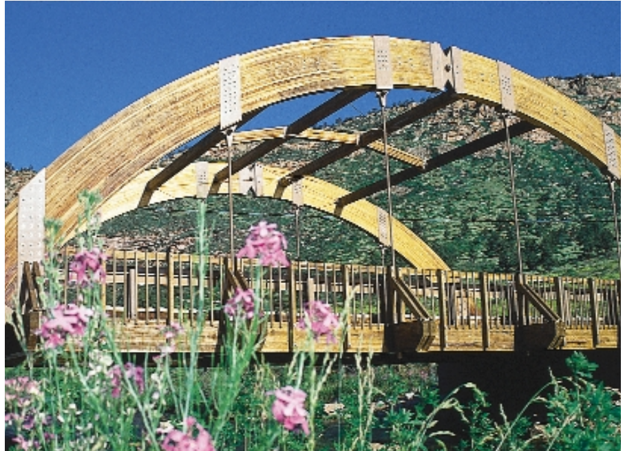
Two lane highway bridge in Colorado using glulam radial arches.
