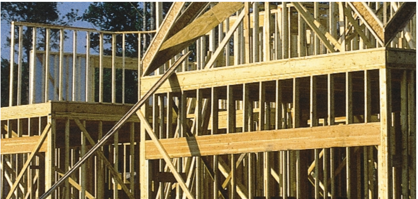
Glulam headers support framing in this two-story home.
