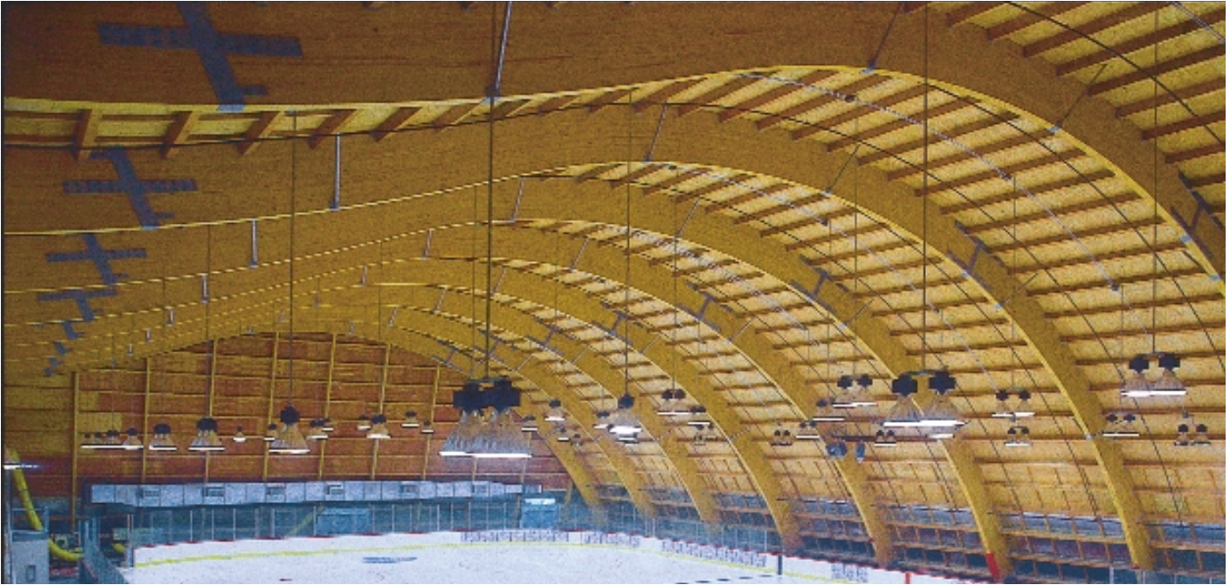
The Disney ICE rink in Anaheim, California features glulam arches curved to a 75-foot radius to form the ice center's roof system.
