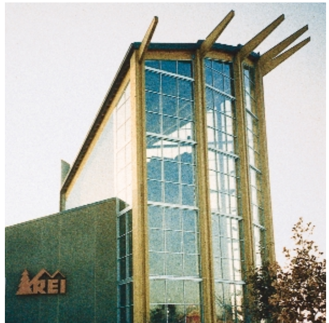
REI, an outdoor sports equipment retailer, used glulam columns and beams in its Minneapolis, Minnesota store.
