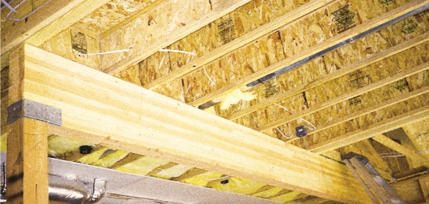
Glulam beam supports second floor I-joist construction.
