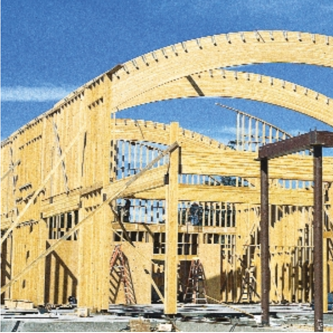
Curved beams define the building design in the Steinbeck Center, Salinas, California.
