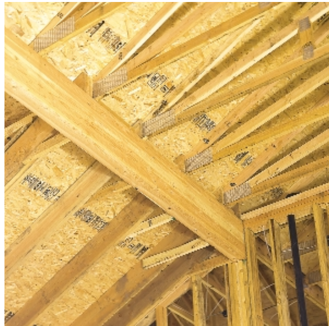
Glulam ridge beams complement the spacious, open designs common in modern residential construction.
