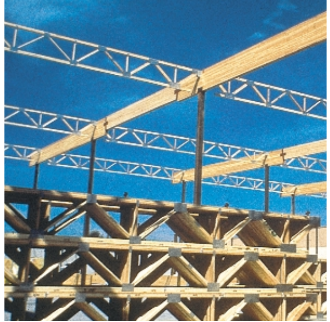
Panelized wood roof with open web glulam trusses and beams.
